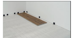
Figure 1: Planks should be staggered, with at least 8" (200 mm) or 25% of the length of the plank between end joint of adjacent planks. No plank less than 6" (150 mm) should be installed. Stagger planks to avoid installing in a brick like pattern on alternating rows. It is very important that the first two rows are installed properly. Installation will alternate back and forth between rows one and two, for the first two rows only. The first row of planks will be placed with the grooved edge facing outward into the room.
