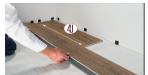
Figure 3: Use a full-length board for Plank 2 which will be installed in the second row. Align plank 2 at an angle, onto the long side of plank 1 making sure there are no gaps. Drop plank 2 to lock in place.
