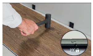
Figure 7: Continue alternating planks on rows 1 and 2. Ensure planks are properly aligned along the chalk line and against the spacers. Finish rows 1 and 2 in this manner, cutting planks at the end of the row, as necessary. Ensure that the end planks are a minimum of 6" (150 mm) in length. If necessary, adjust the length of starter pieces to insure minimum plank lengths for each row, with proper end joint stagger row to row.
