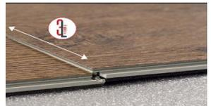
Figure 6: Using a rubber mallet, lightly tap the joint on the short side to engage the locking system.
