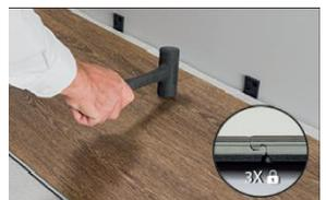
Installation of all additional rows will start by angling a plank on the long side and sliding plank to the left until the short sides are in contact. Lock the short side as instructed for rows 1 and 2 using a rubber mallet to engage locking system as shown in Figure 5.
