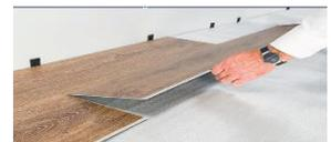
Figure 7: Continue alternating planks on rows 1 and 2. Ensure planks are properly aligned along the chalk line and against the spacers. Finish rows 1 and 2 in this manner, cutting planks at the end of the row, as necessary. Ensure that the end planks are a minimum of 6" (150 mm) in length. If necessary, adjust the length of starter pieces to insure minimum plank lengths for each row, with proper end joint stagger row to row.
