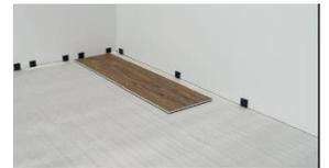
Figure 3: Use a full-length board for Plank 2 which will be installed in the second row. Align plank 2 at an angle, onto the long side of plank 1 making sure there are no gaps. Drop plank 2 to lock in place.
