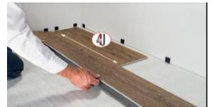
Figure 4: Working from the wall, insert plank 3 into the long side of plank 2.
